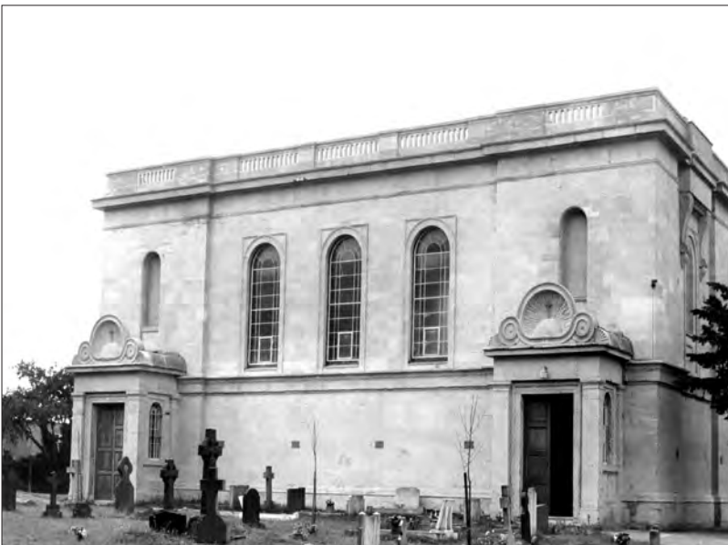
The church looked like this in 1966 after the removal of the bell tower. The removal of the graveyard fence probably took place during WWII. Photo : Centre for Oxfordshire Studies - D-266685a.
